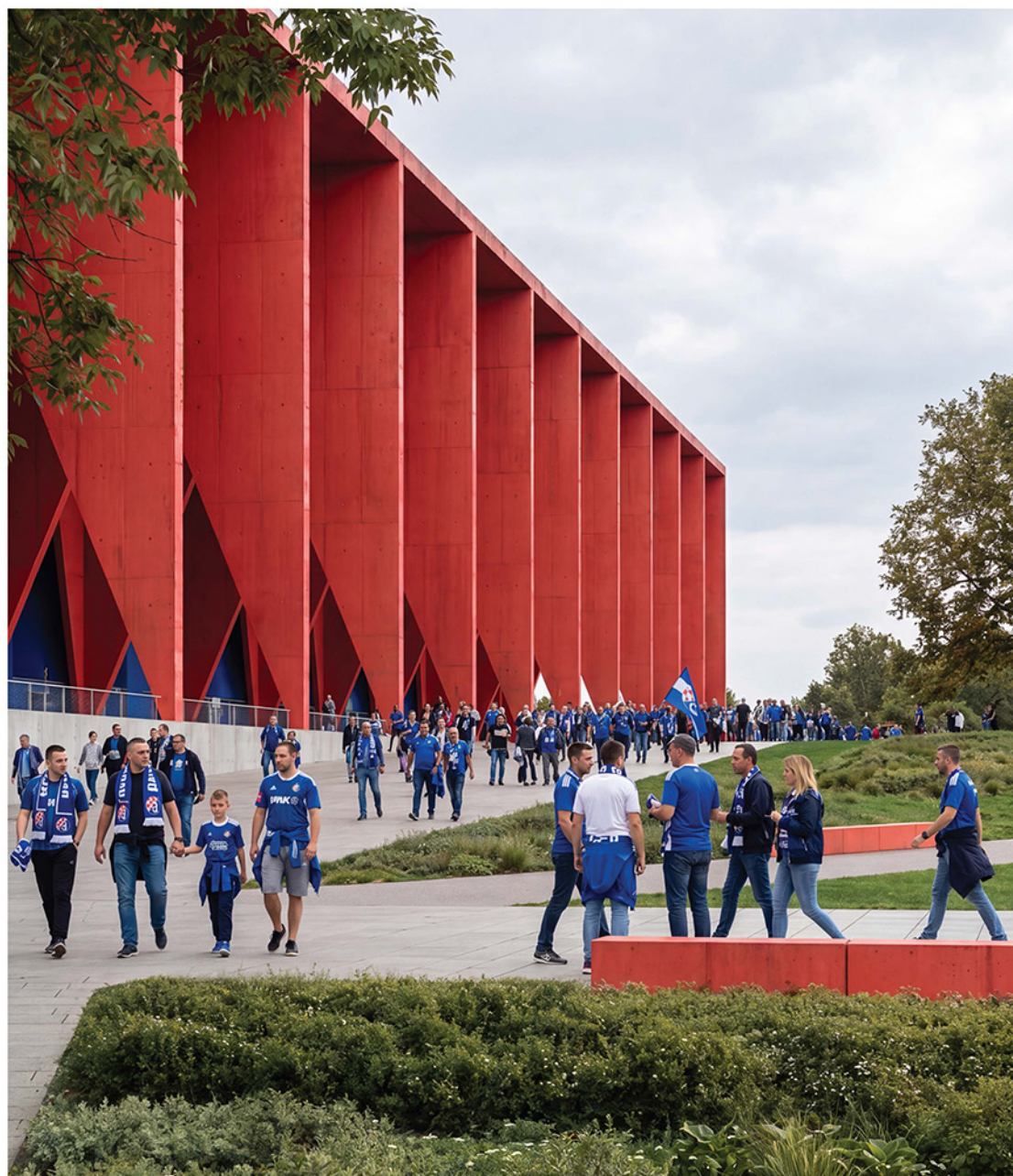
View of the north-west entrance zone
