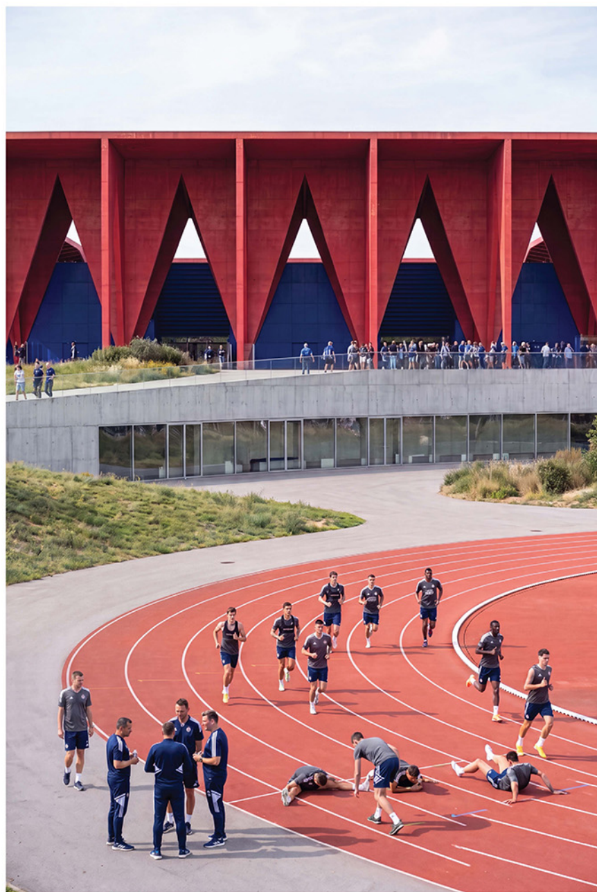
View of the Athletics stadium zone
